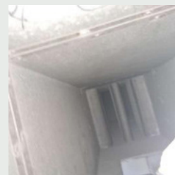
Down the Duct (Duct condition)
